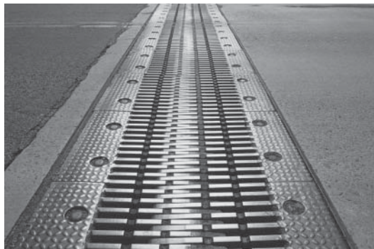
(b) Bridge expansion joint
